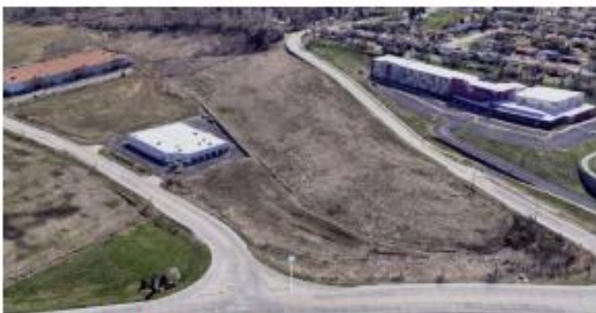
Mills Mall Hill, Looking West
